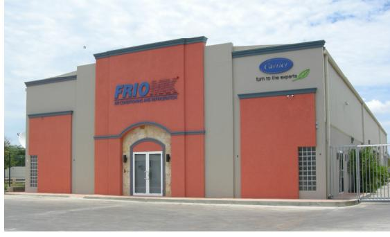
store, consists of 9600 sq. ft. of storage, office, and retail space. It features a full height block parapet wall at the storefront. The remaining walls combine block with Dean's Rib-12 Light Stone panels. The roof received 24 ga. Rib-12 Oyster White panels. Dean also provided a 60' x 60' complete mezzanine system for the building.
