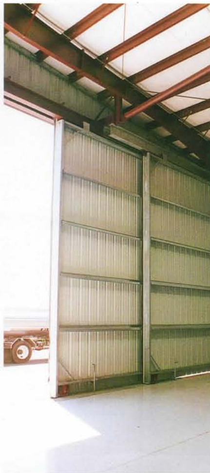
Standard Corporate Door & Wheel System. Shown is optional Galvanized Stiles & Girts.
