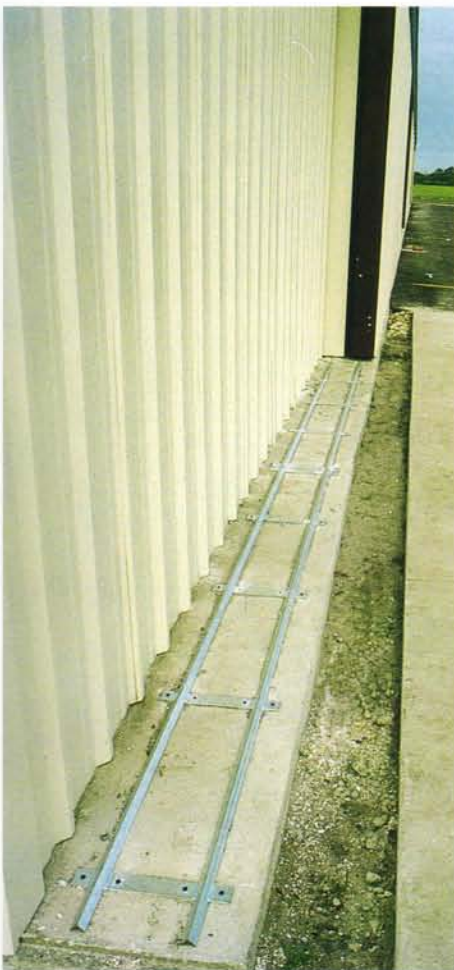
Inverted Angle T-Hangar type track. Shown is optional Galvanized Track.
