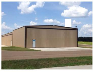
Our first job for Barnard & Sons Construction, Mendenhall, MS. is a six-unit bi-fold nested T-Hangar with a 50 x 50 bi-fold jet pod on one end. DSB provided a smoother appearance by offering to increase the jet pod width to 52' to match the T-Hangar. The hangar is located at Copiah County Airport in Hazelhurst, MS.
